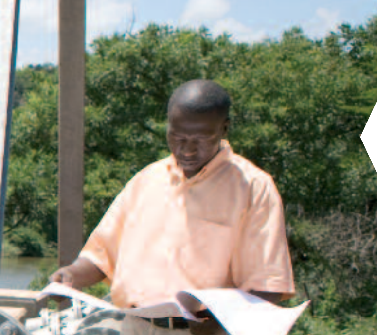
A District Official conducting a site inspection of a Ekulindeni new pump station at Albert Luthuli Municipality.
